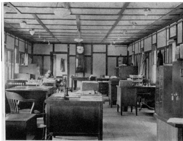
Interior of the old main office.
